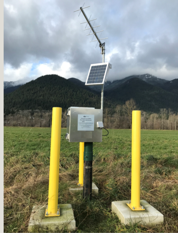
A provincial OW site with a data logger & telemetry
