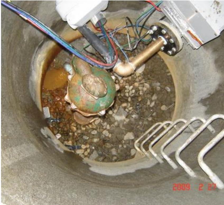
**Must not construct well pit for new/altered water supply wells**
