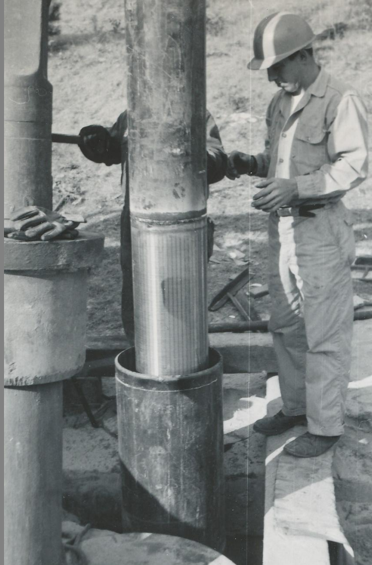
Installing a well screen.
