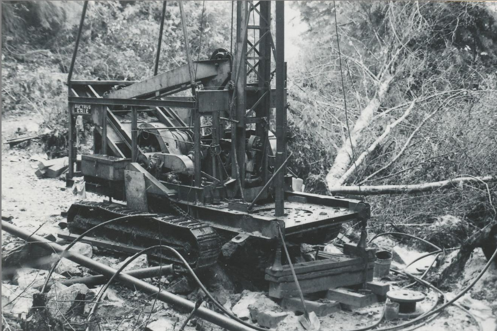
Blast hole rig used to drill a well in Bamfield
