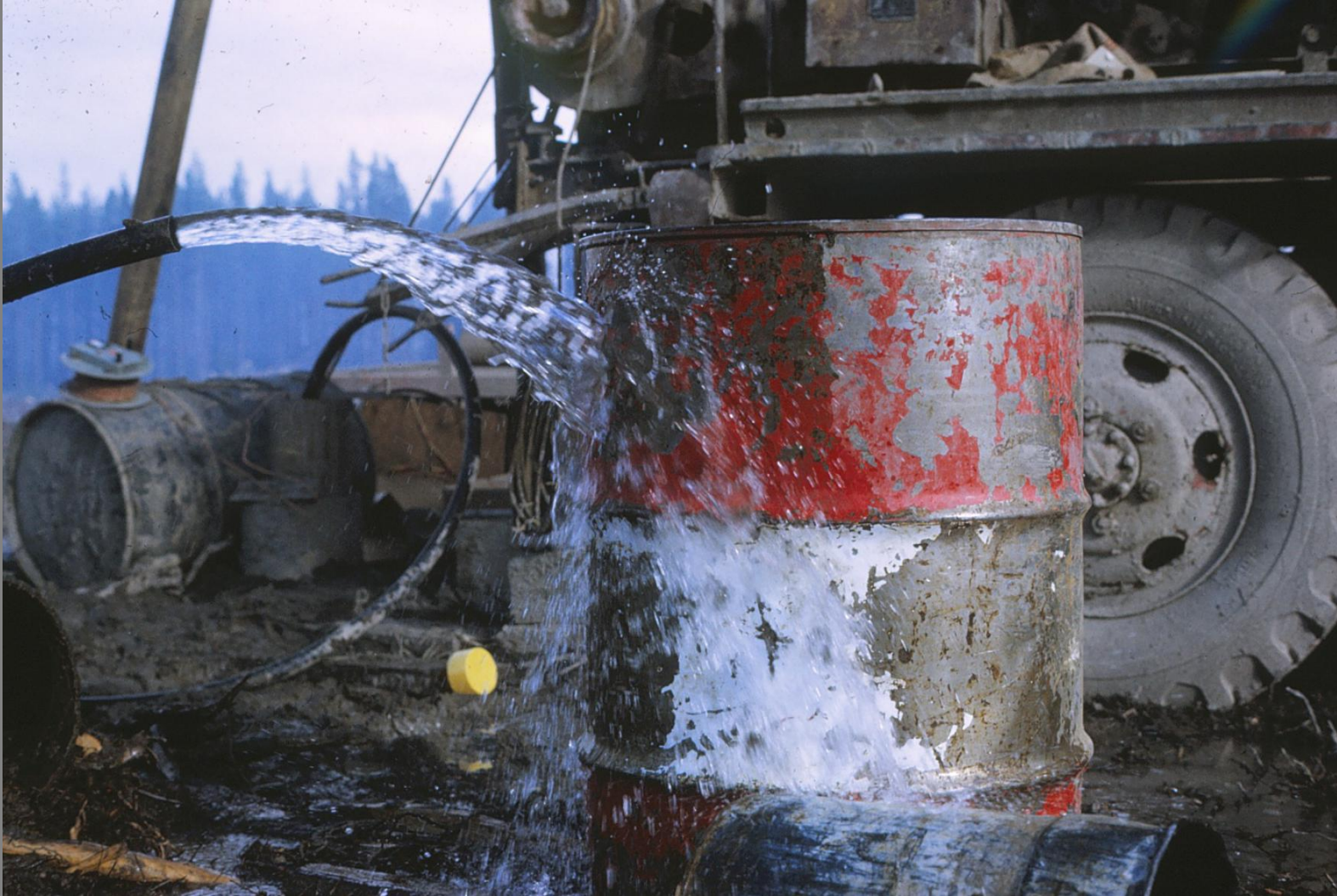
30gpm discharge from completed 40m deep Takla mill well
