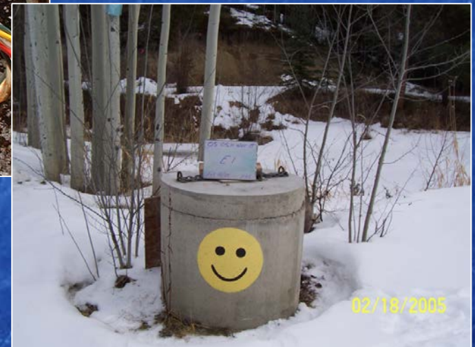
Concrete lid on dug well
