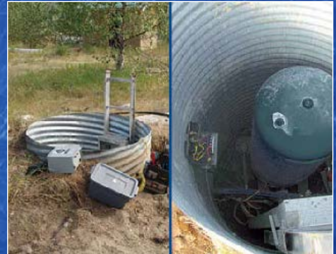
Drilled Wells in Pits
