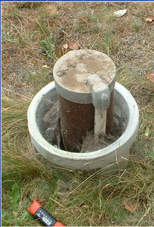
Cap with space for wiring (pitless adapter style set-up)
