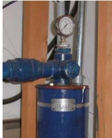
Figure 7. Well head with ID plate.
